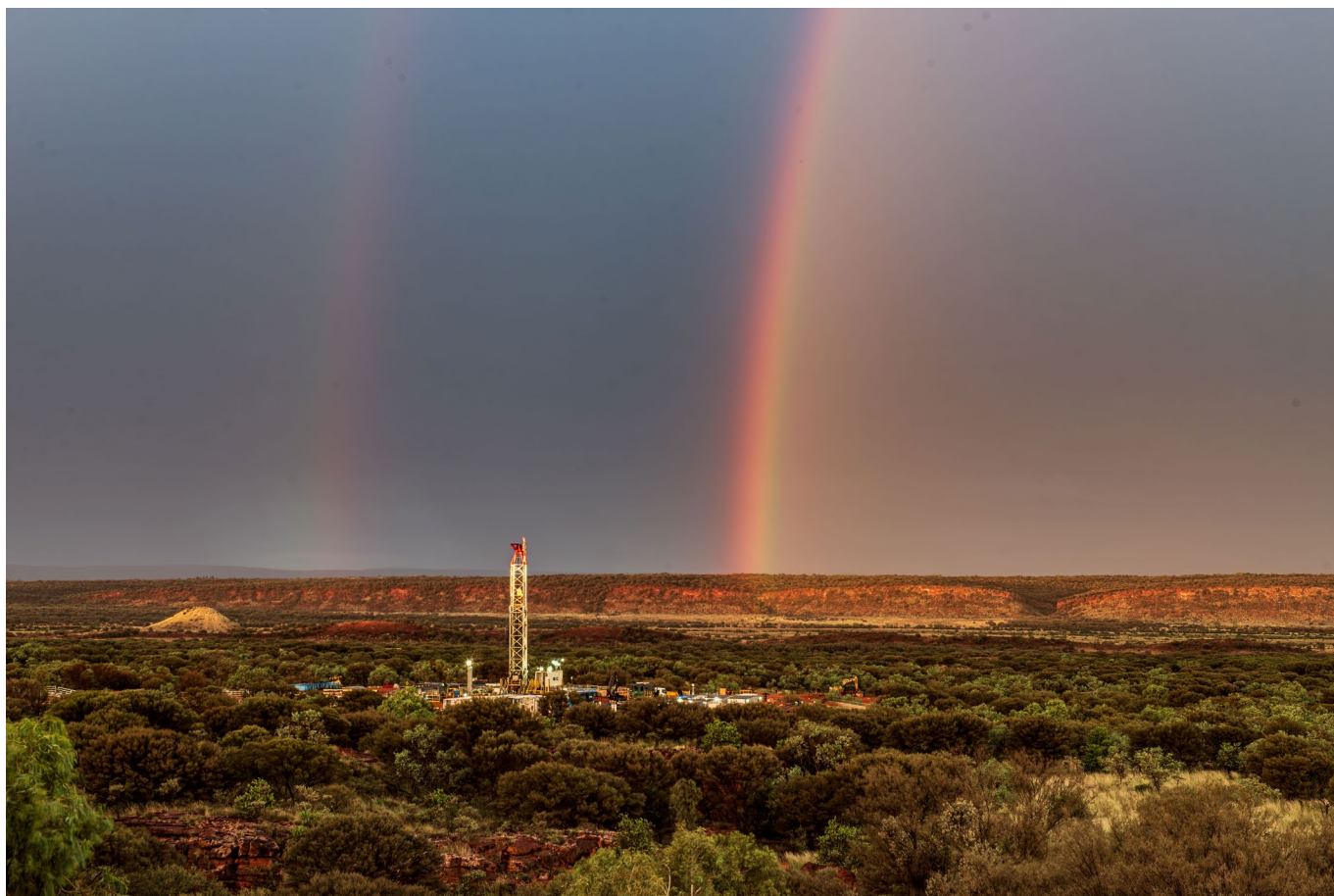
Drilling rig at Mereenie
