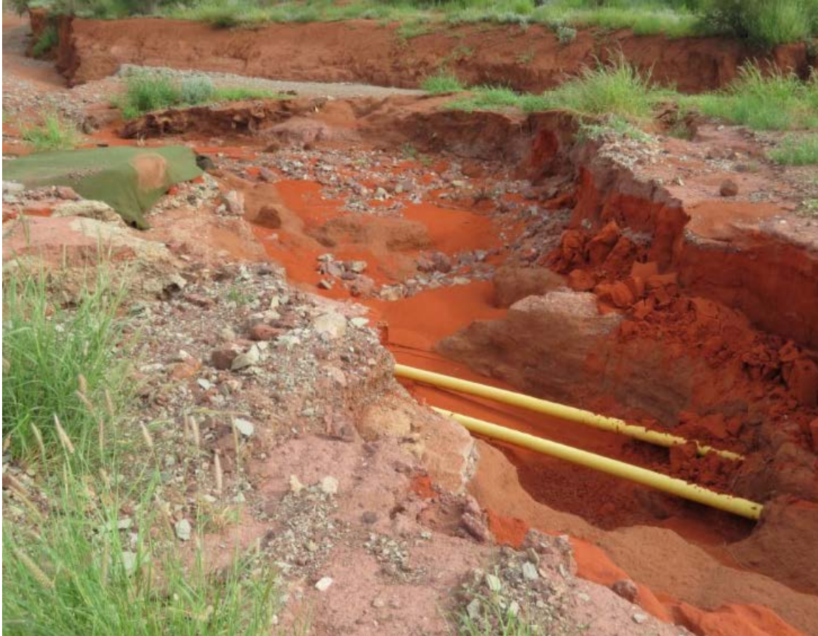
Figures 2 & 3: BEFORE: ESS access road - exposed gas pipeline at the culvert caused by erosion.
