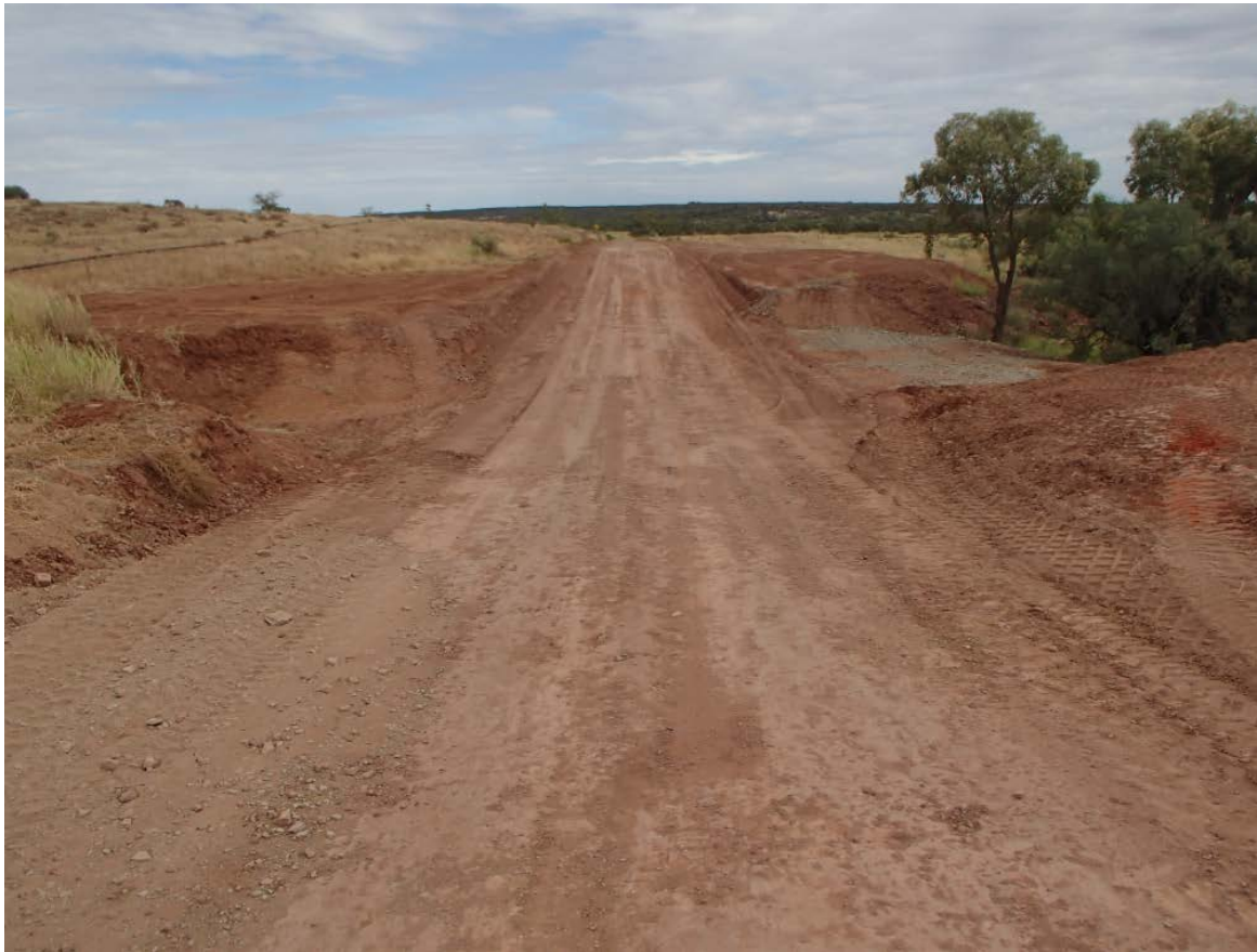
Figures 4 & 5: AFTER: Culvert has been removed. Road taken down to the creek level. Pipe has been reburied.
