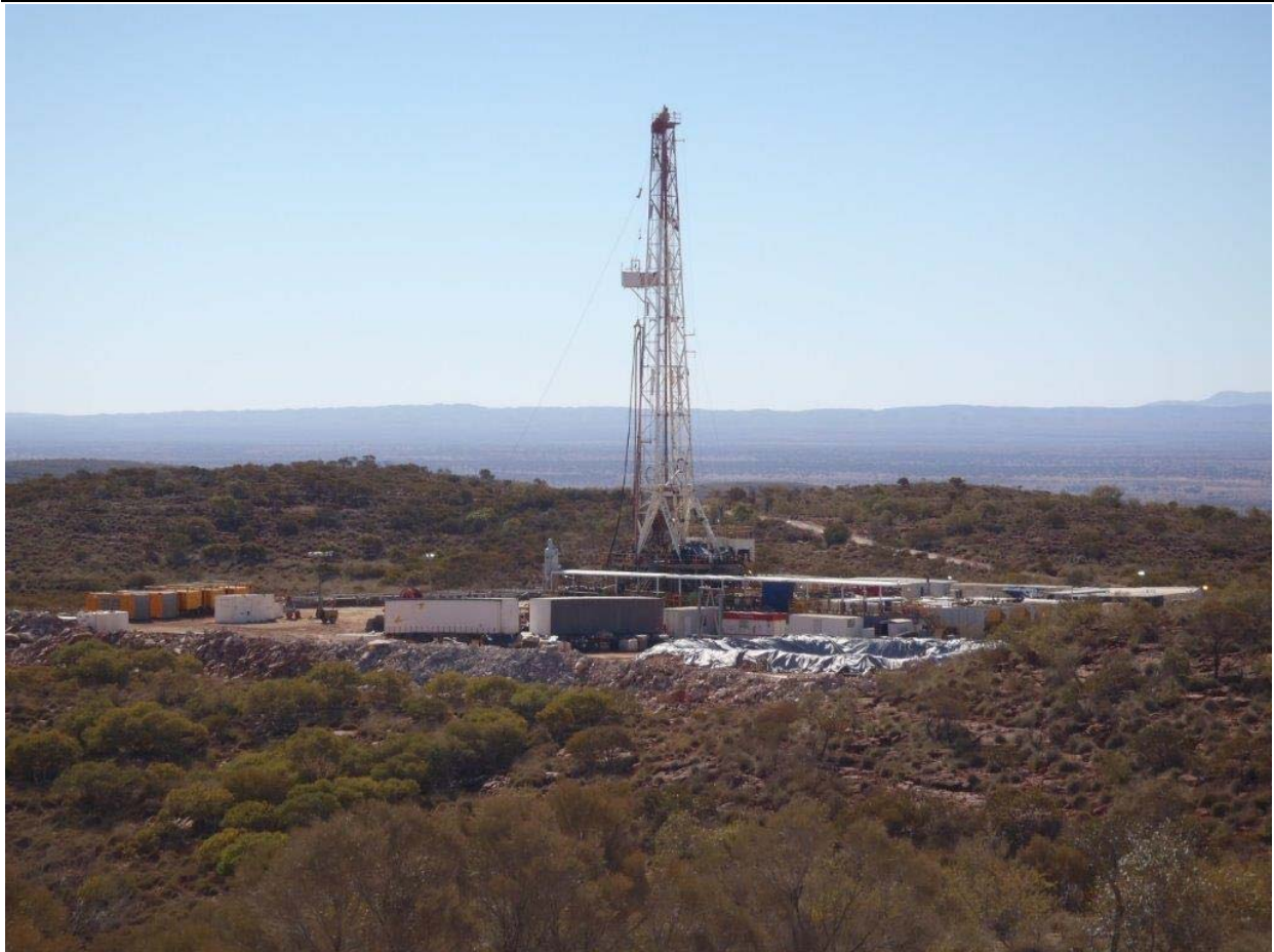
Figure 1: Rigged up and Drilling at Palm Valley 13
