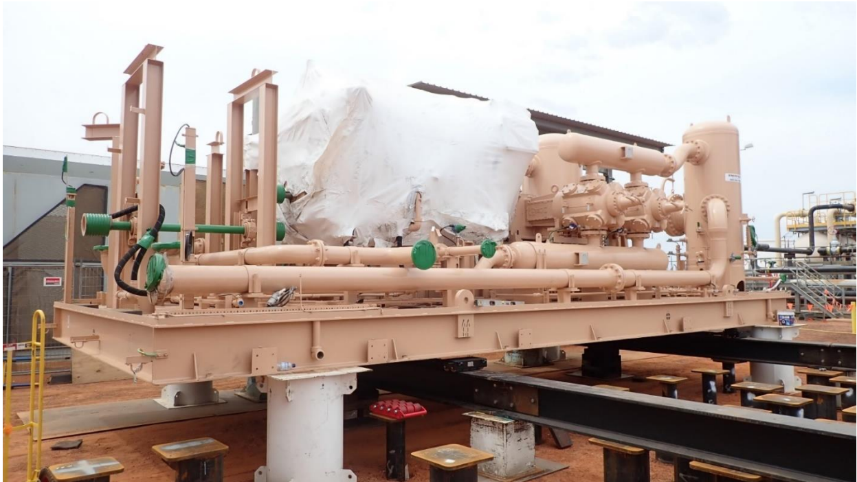
Figure 1: Installation of the new Field Boost Compressor at Mereenie
