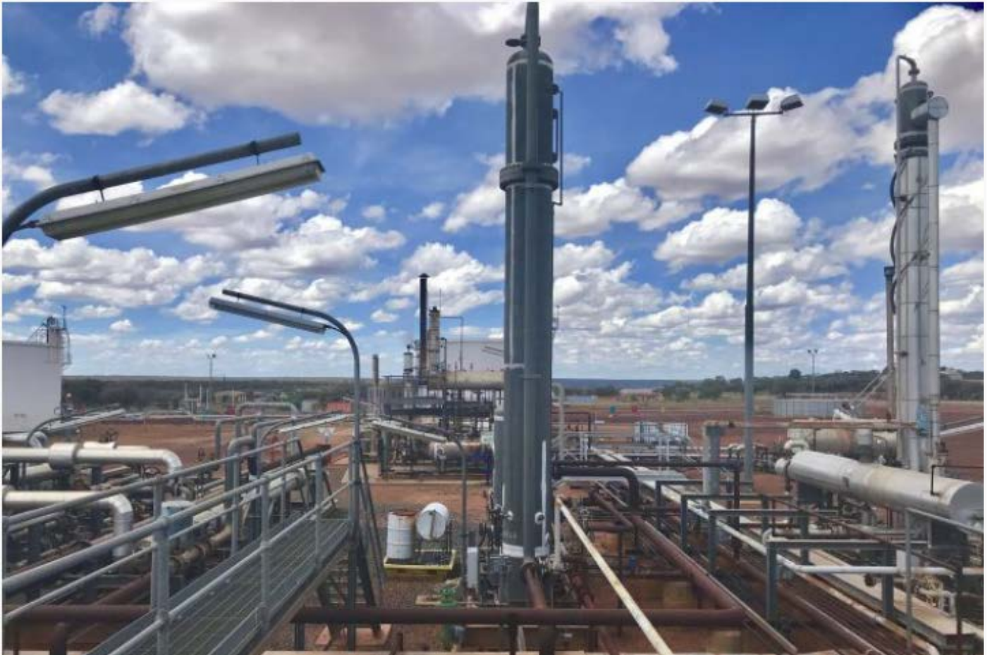
Oil, gas and water from the Mereenie field's wells are separated and processed at Central Petroleum's plant on site. (ABC Rural: Katrina Beavan)
