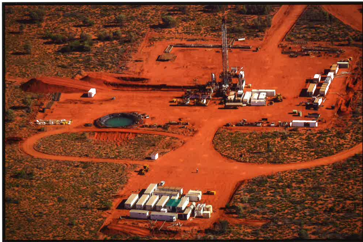
An aerial view of Central Petroleum's Surprise-1 site, Northern Territory. (Source: Central Petroleum)
